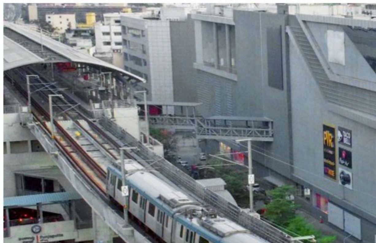
A skywalk linking the Punjagutta Metro station to a mall.
