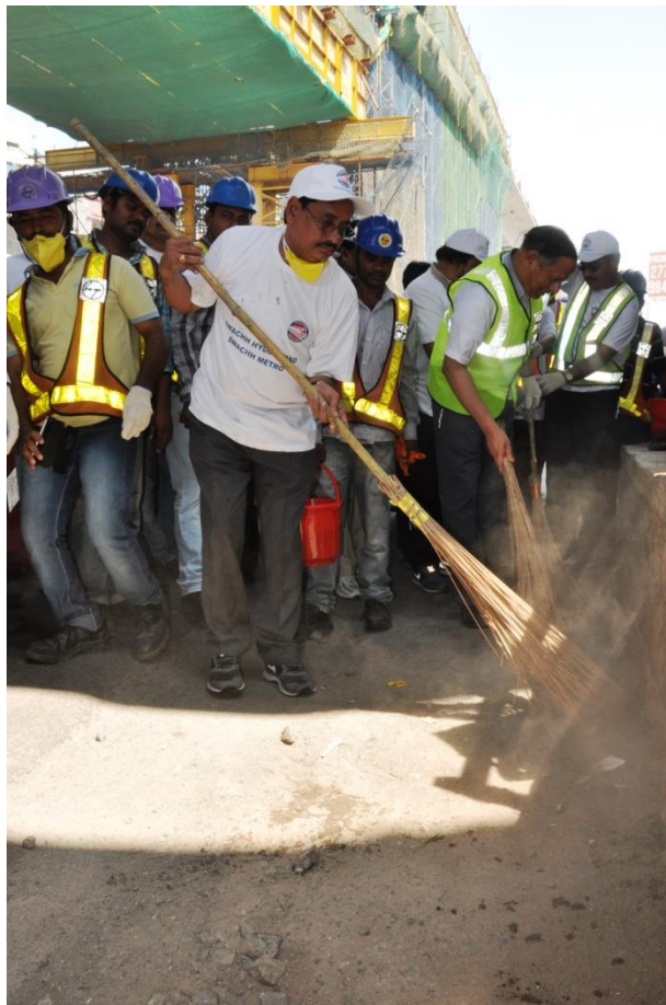
MD, HMR Mr.NVS Reddy cleaning the Metro construction site at Punjagutta on Sunday (May 17, 2015)
