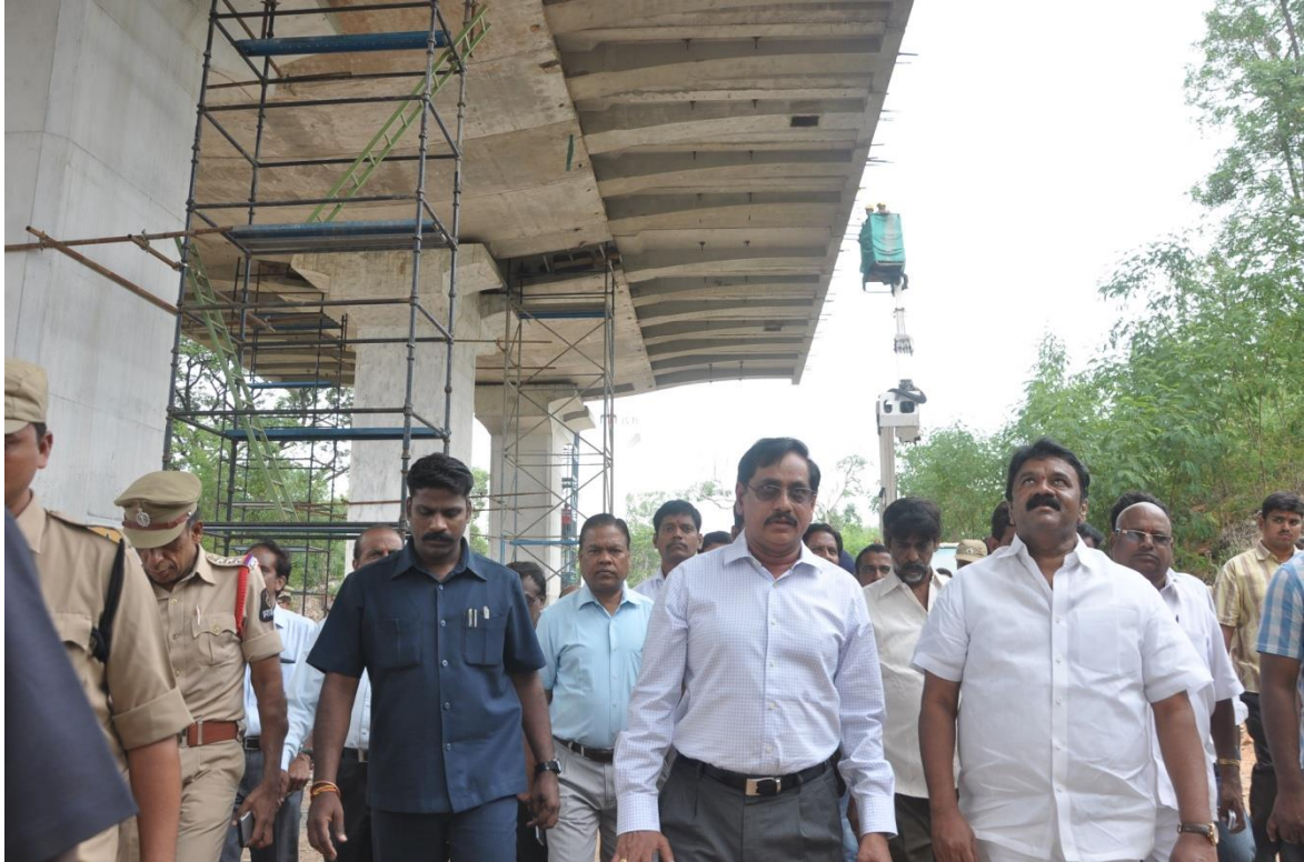
Minister for Commercial Taxes and Cinematography Mr. Talasani Srinivas Yadav and MD, HMR Mr. NVS Reddy inspecting Secunderabad (East) Metro Rail station construction activity of corridor-II in Old Gandhi hospital premises on Thursday (July 30, 2015)
