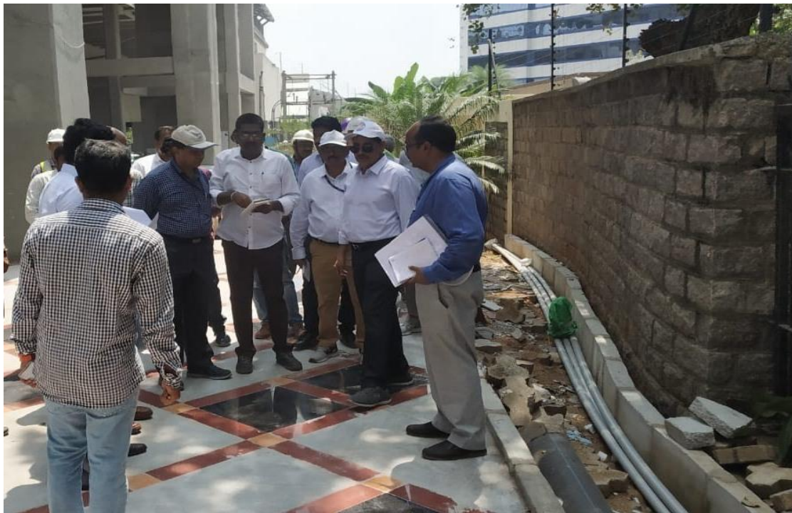
MD, HMRL Mr.NVS Reddy along with HMRL engineers inspecting Urban Rejuvenation works at Hitec City Station on Sunday (30.09.2018)
