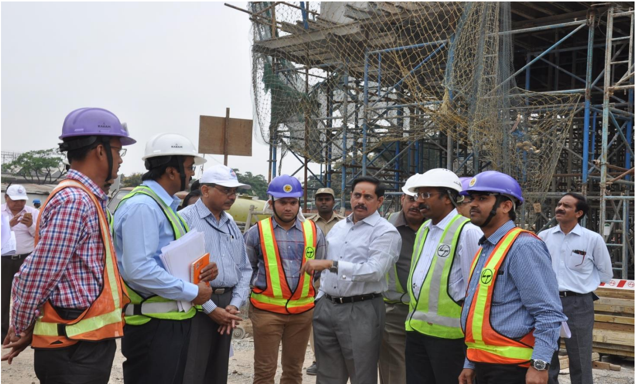
MD, HMR Mr. NVS Reddy advising engineers of HMR and L&TMRHL during his inspection at Metro Rail interchange station at Imlibun on Monday (November 16, 2015)
