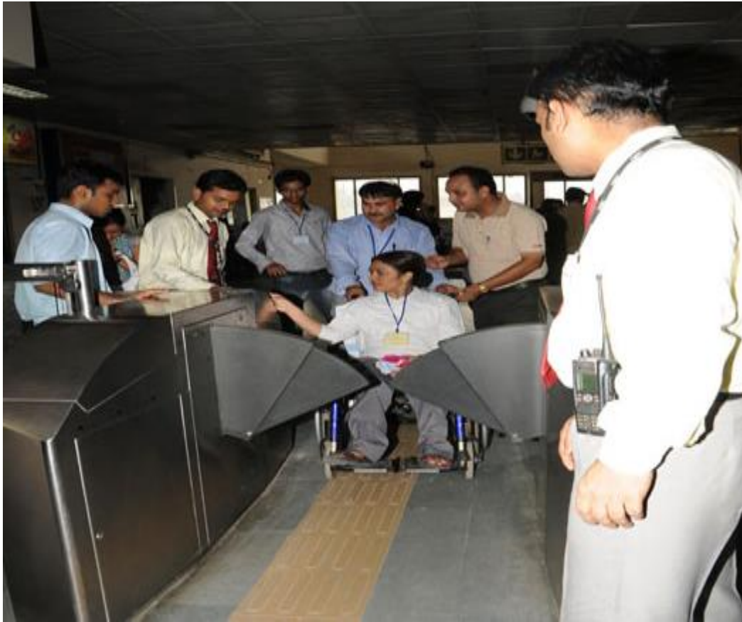
Figure 3: Wide Automatic Fare gates for wheelchair passengers
