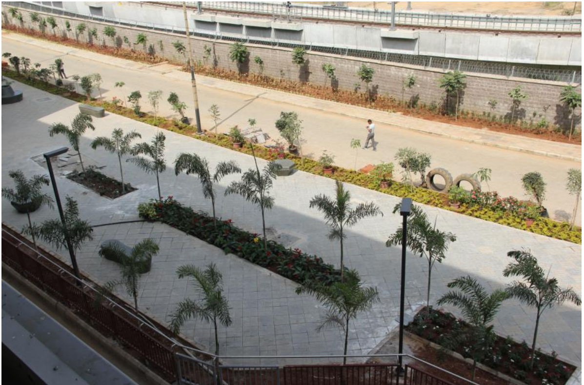
Miyapur urban rejuvenation works in progress
