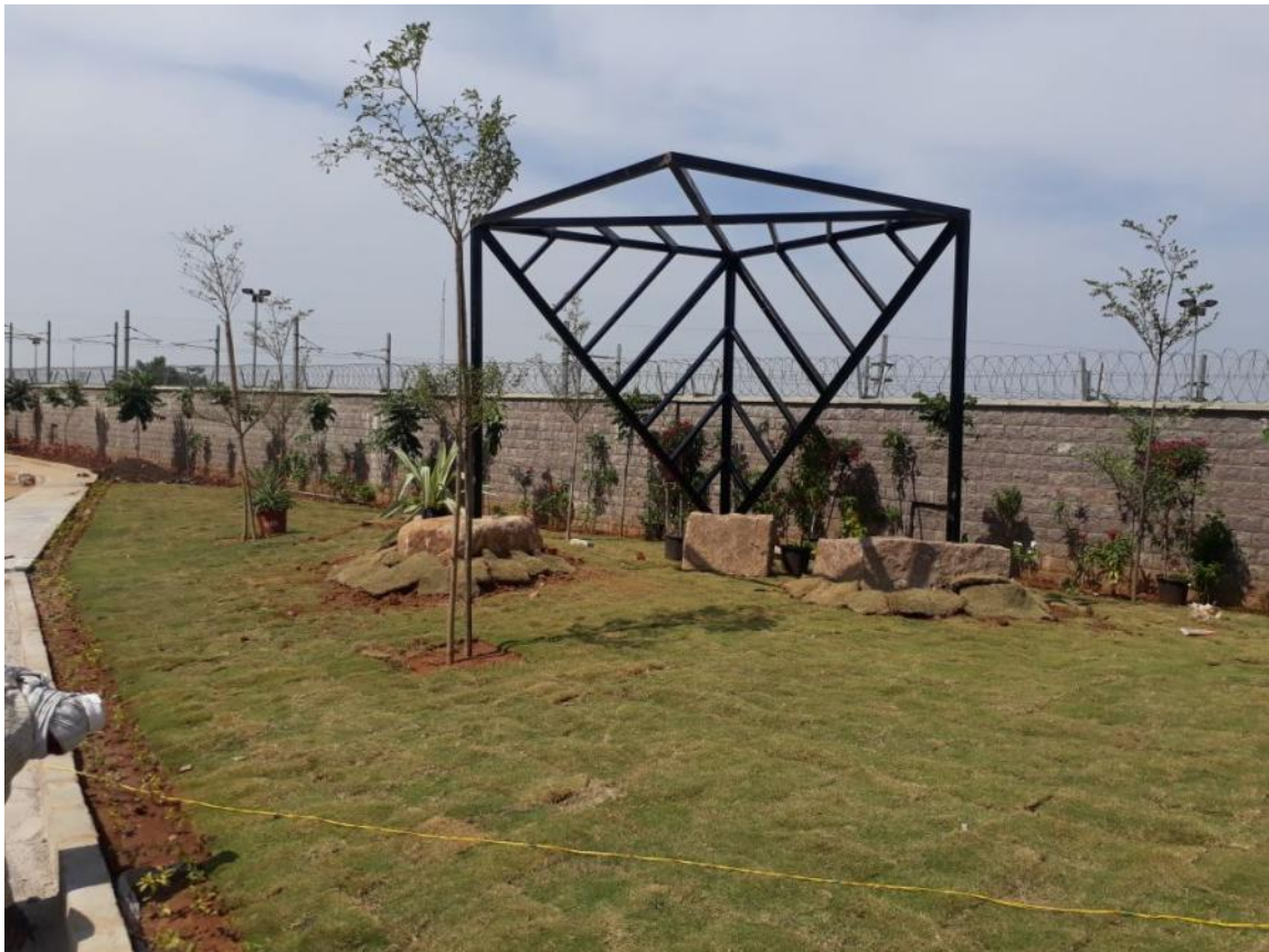
Miyapur urban rejuvenation works in progress
