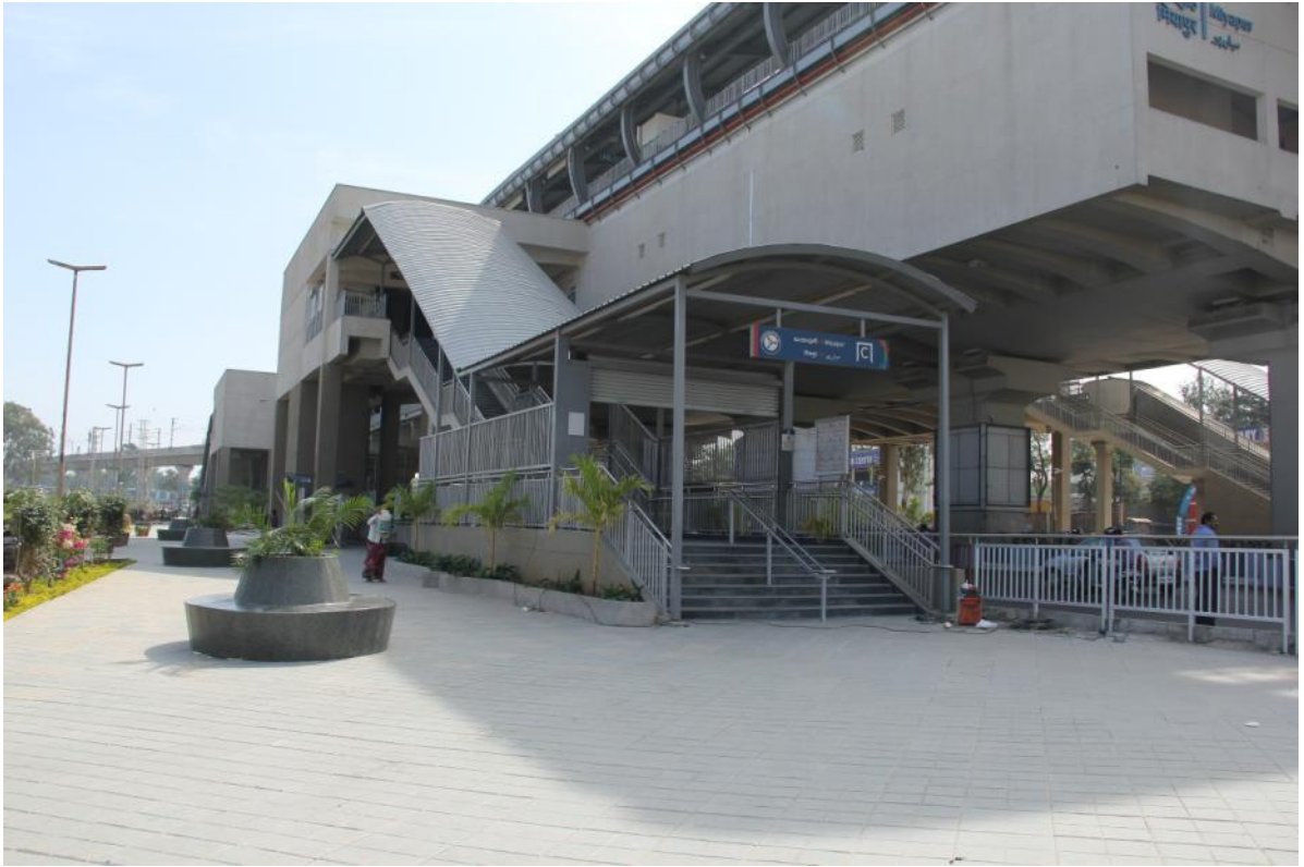
Miyapur urban rejuvenation works in progress
