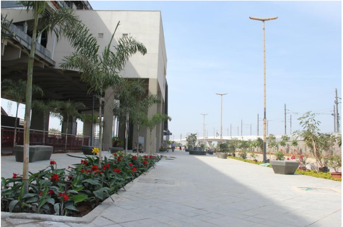
Miyapur urban rejuvenation works in progress
