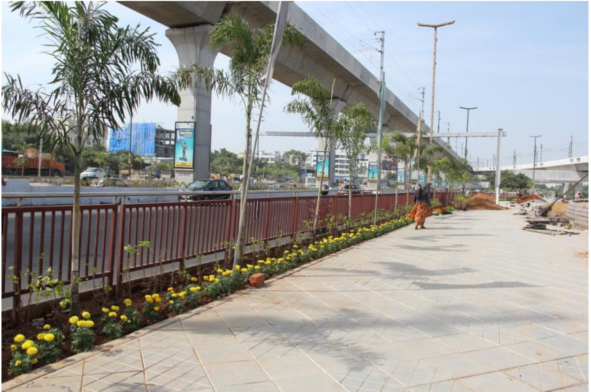
Miyapur urban rejuvenation works in progress
