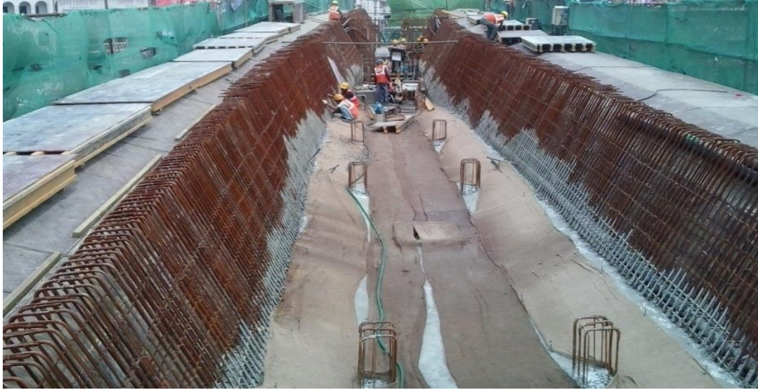
Bottom slab work completed for cast In-situ span (during construction)
