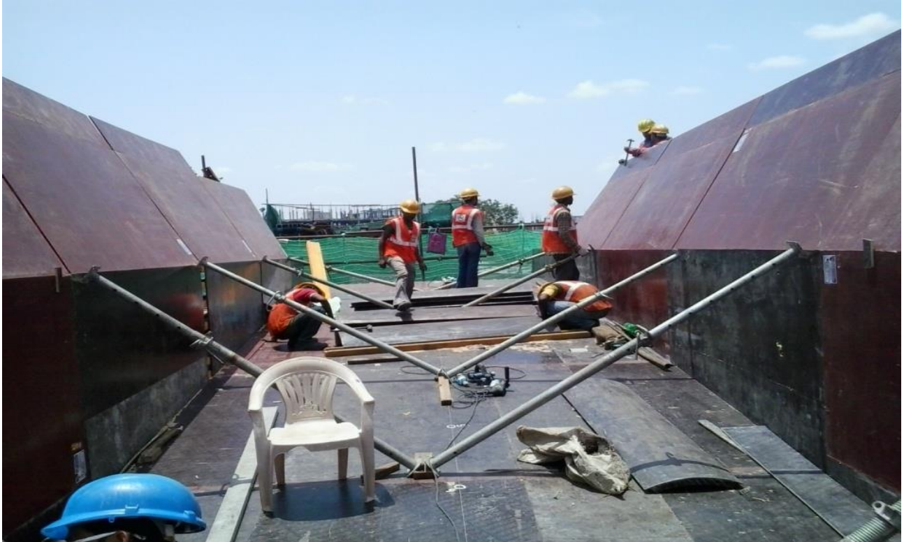
Shuttering in progress for cast In-situ span (during construction)
