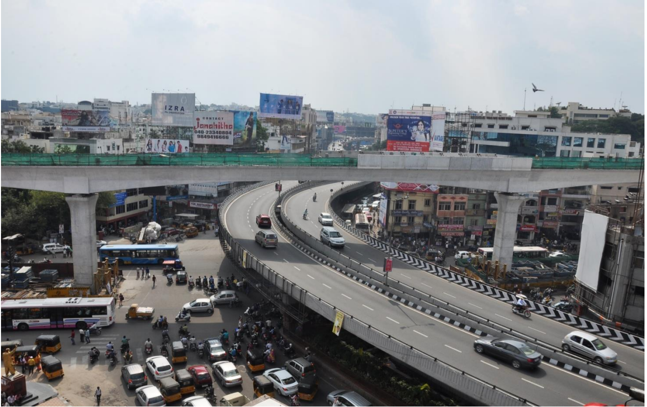
Aesthetic and iconic Metro viaduct crossing the existing flyover at Punjagutta
