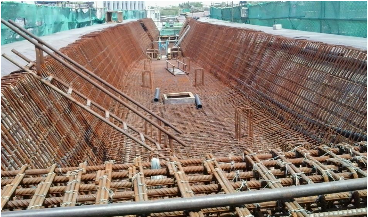
Reinforcement work in progress for cast In-situ span (during construction)
