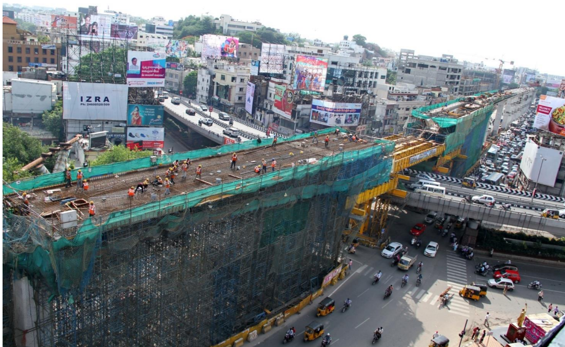
Formwork arrangements for three spans continuous at Punjagutta Cast In-situ
