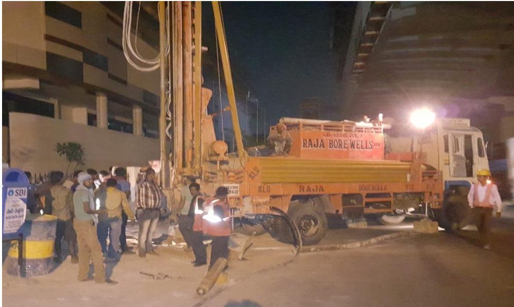
Borewell drilling for construction of RWHS near Institute of Engineers, Khairatabad
