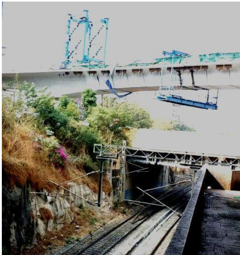
A view of Metro ROB above MMTS at Lakdi-ka-pul
