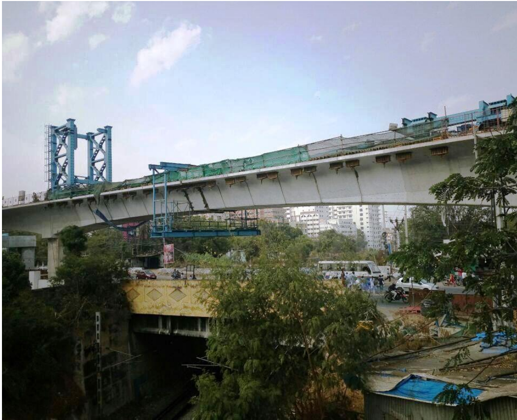
Completed view of Metro ROB using 'Bridge Builder' at Lakdi-ka-pul
