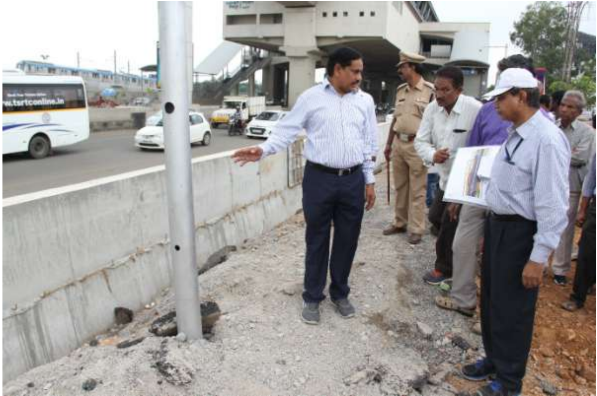
MD, HMRL Mr. NVS Reddy inspecting service road formation and other urban rejuvenation works at Miyapur Metro station on Monday (02.10.2017)
