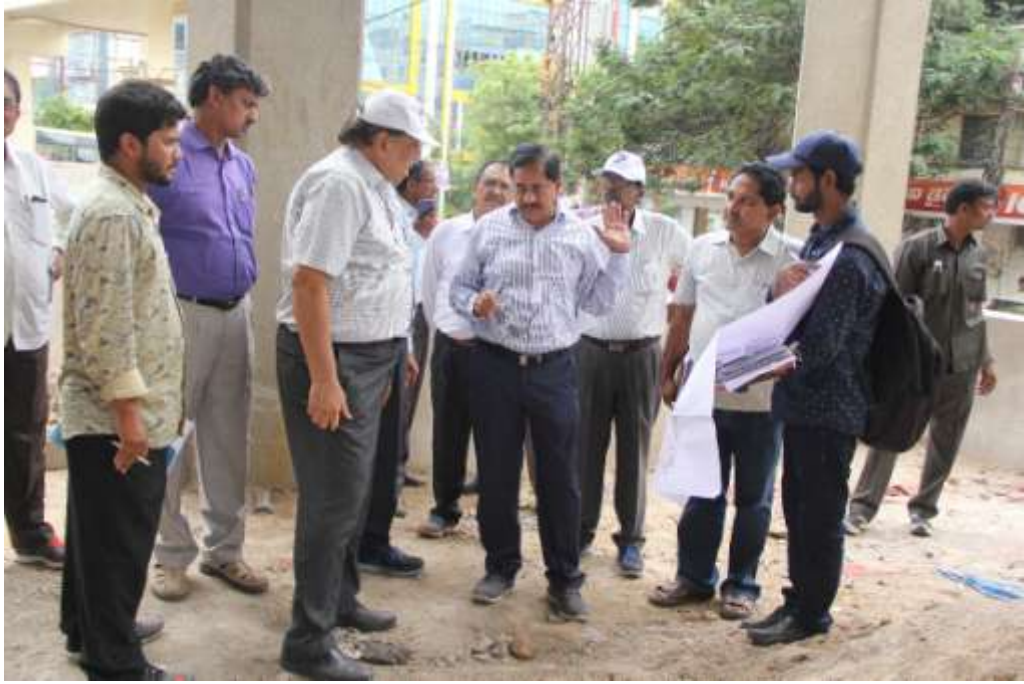
MD, HMRL Mr. NVS Reddy giving instructions to HMRL engineers on urban rejuvenation works at KPHB Metro station on Monday (02.10.2017)
