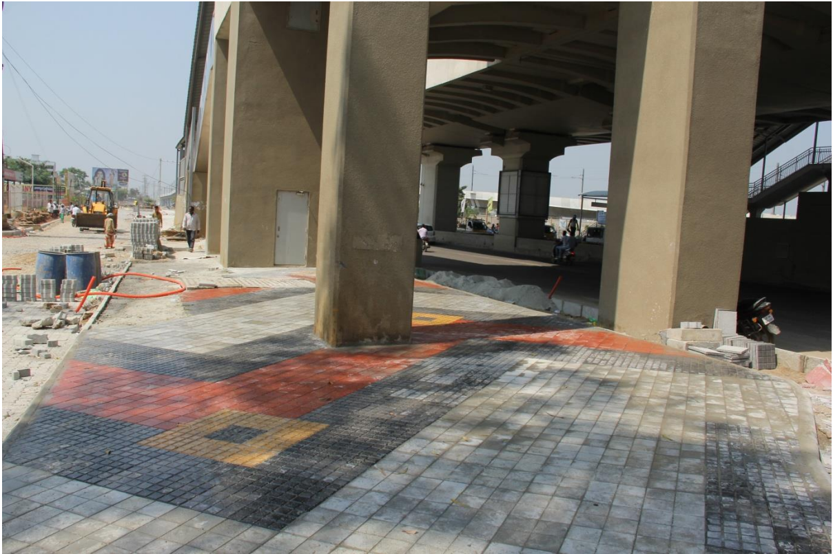
Miyapur station works in progress
