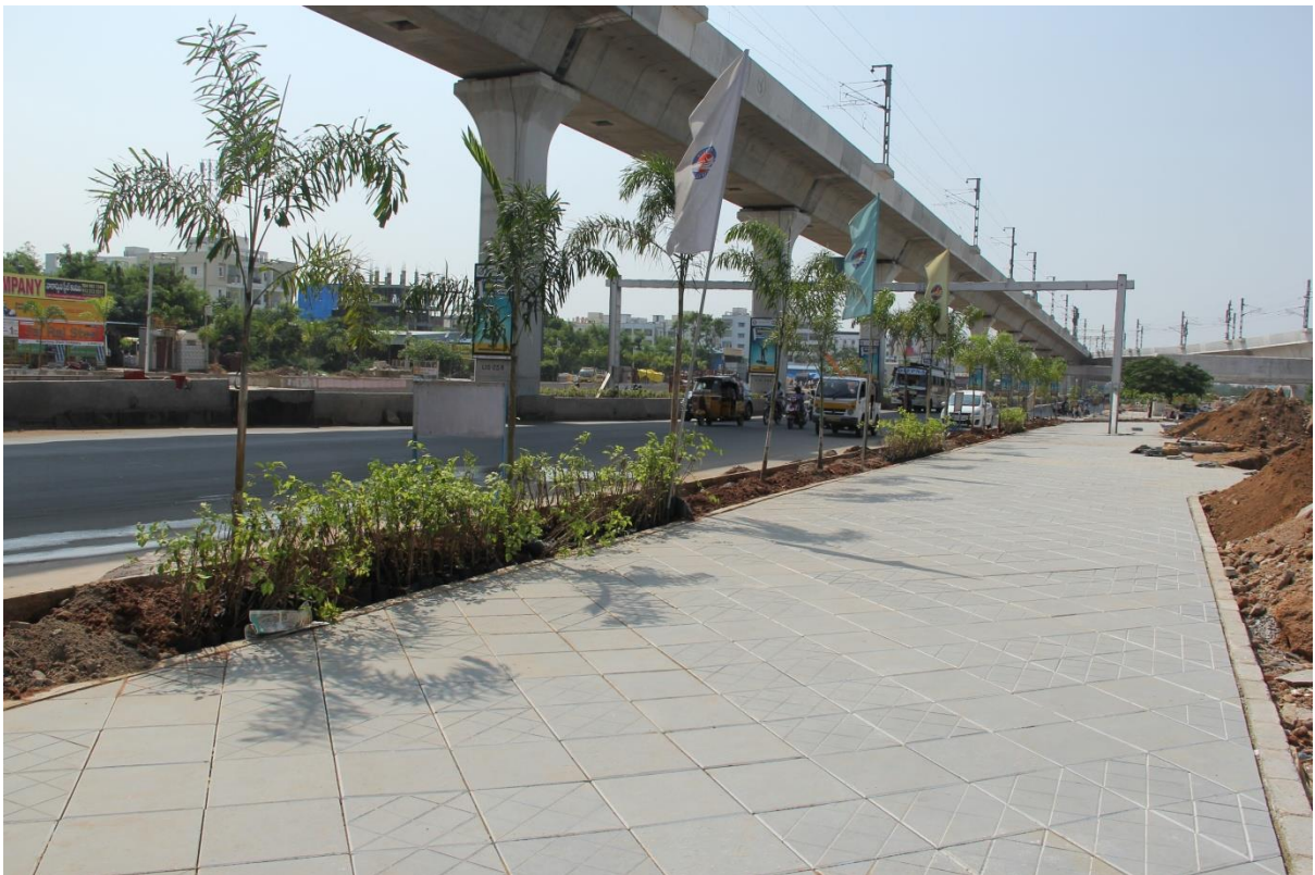
Miyapur urban rejuvenation works in progress
