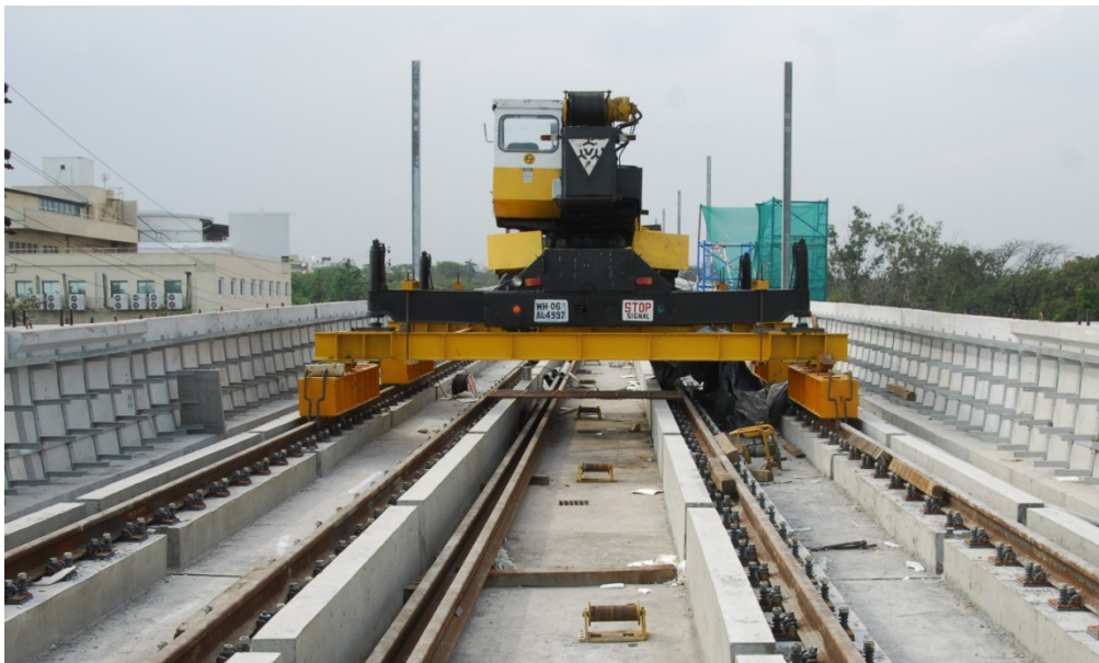
Track Master- A unique instrument for high accuracy of Track parameters and enhancing the quality of track installation.
