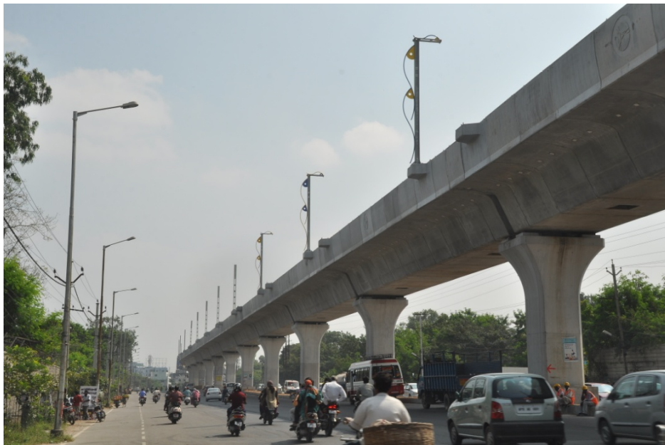
Aesthetic construction of Hyderabad Metro Rail elevated viaduct.
