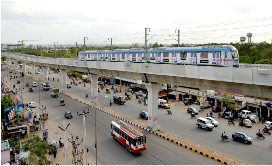
Test run of Hyderabad Metro train on viaduct.
