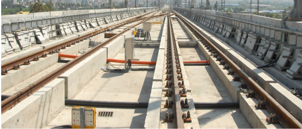
Head-hardened rails for the tracks on the viaduct of Hyderabad Metro Rail (minimal maintenance & cost efficient in 'life-cycle' costing).
