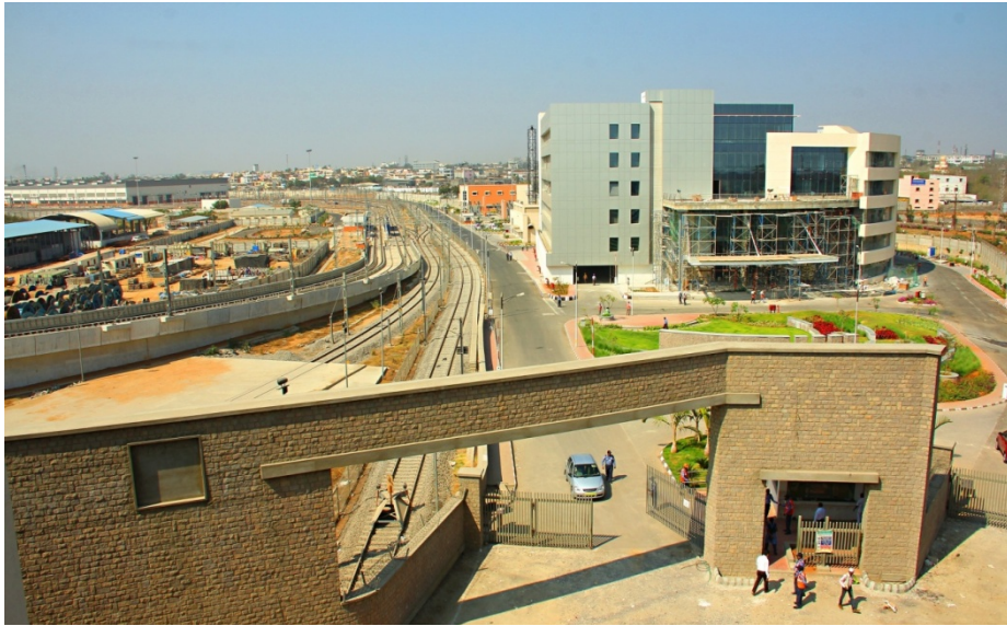
A view of Hyderabad Metro Rail Uppal Depot.
