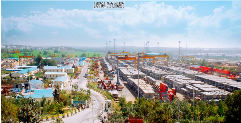
The panoramic view of Uppal precast yard (72 acres- India's biggest urban precast yard).
