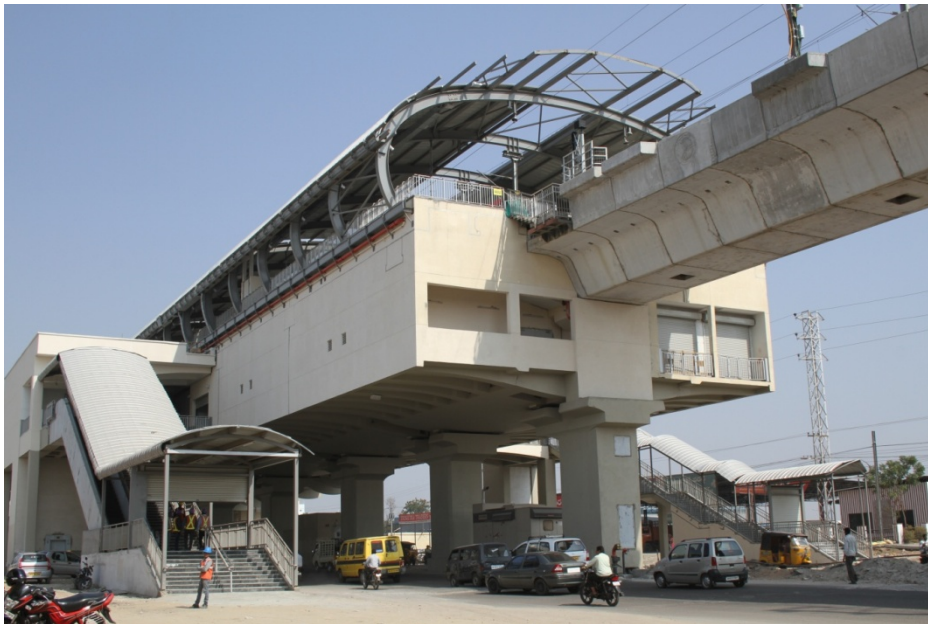
Balanced cantilever Hyderabad Metro Rail station resting on the central piers ('Spine and Wings' prefab construction method – allows free flow of road traffic & avoids 'tunnel' look).
