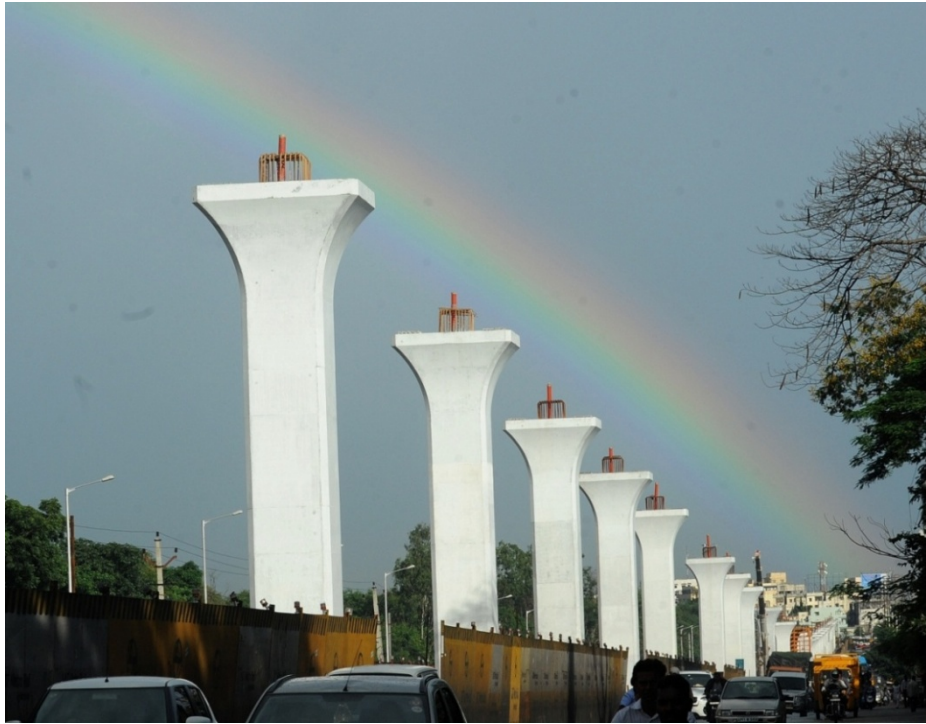
Row of well shaped piers (pillars) of Hyderabad Metro Rail–Aesthetic look.
