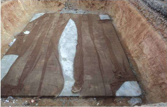
Laying PCC Bed for Foundation
