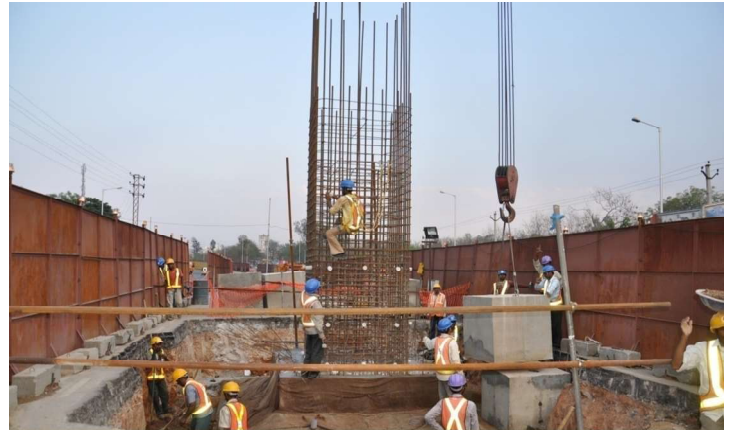
Pier Construction Stage
