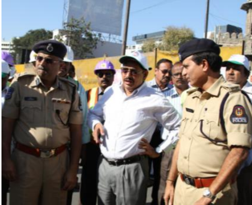
MD, HMR Mr. NVS Reddy conducting inspection with Additional CP (Traffic), Hyderabad Mr. Jitender on road restoration works at MJ market on Saturday (February 07, 2015)
