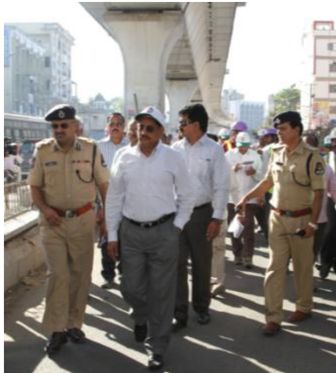
MD, HMR Mr. NVS Reddy conducting inspection with Additional CP (Traffic), Hyderabad Mr. Jitender on road restoration works at Jambagh on Saturday (February 07, 2015)
