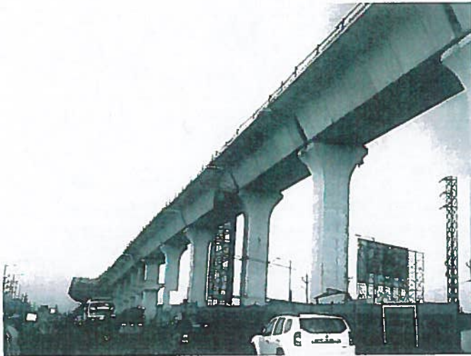
Erected Spans in Stage 1
