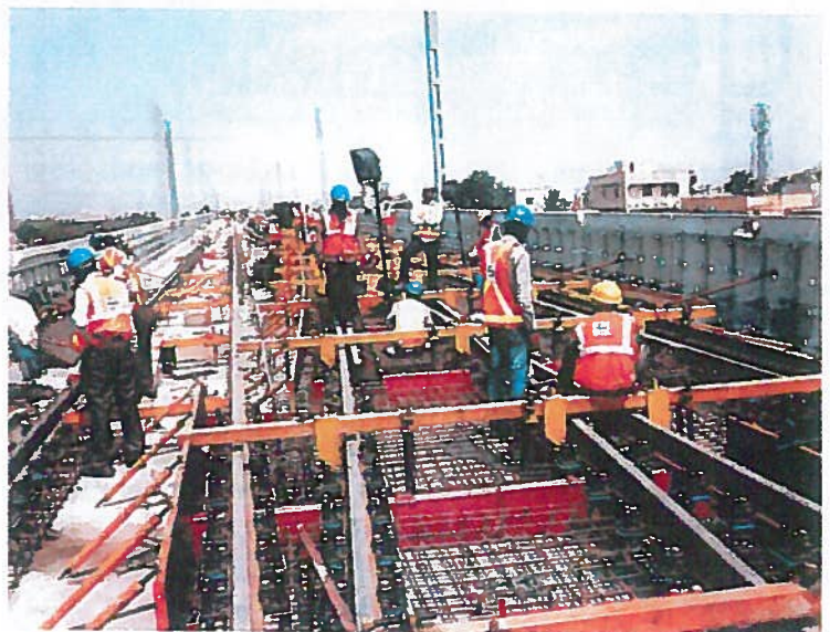
The complex arrangement required for track plinth casting
