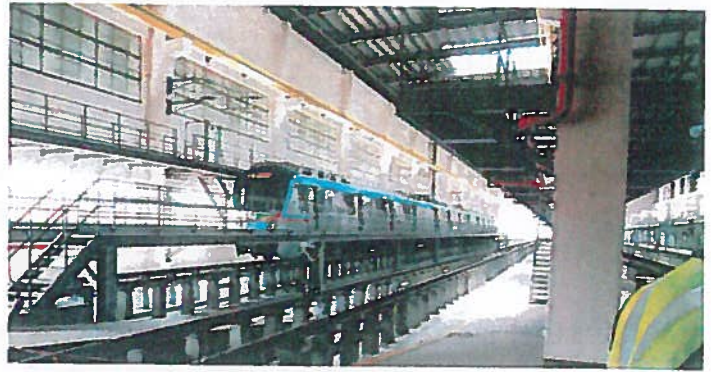
Train set at inspection bay
