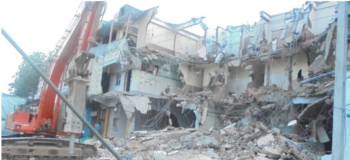
Dismantling of Santosh lodge building at Secunderabad railway station in corridor-II
