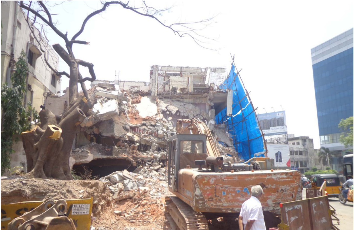
Dismantling of Jabbar building in progress at Begumpet
