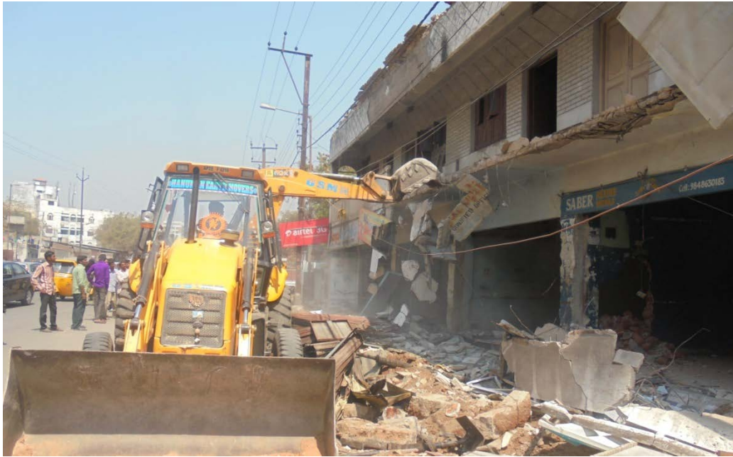
Dismantling of Murali studio building at Musheerabad in corridor-II
