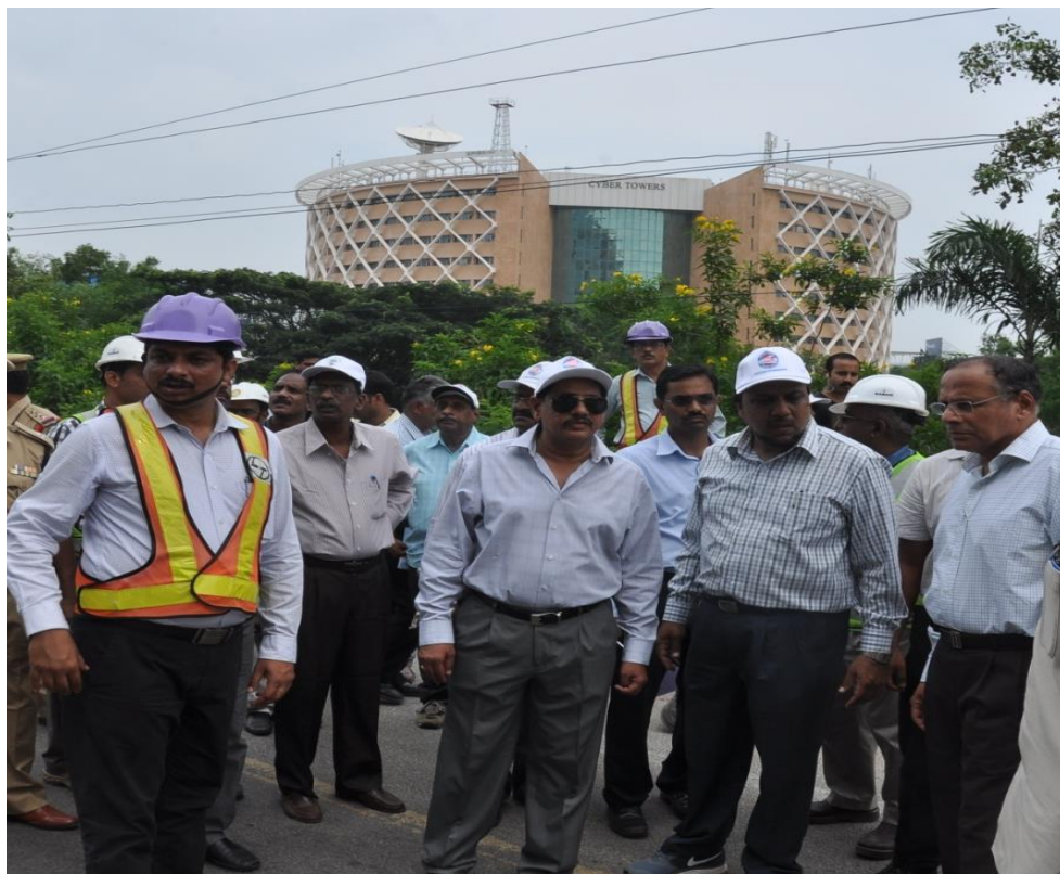
MD, HMR Mr. NVS Reddy inspecting ongoing Metro Rail works near Hi-Tech city
