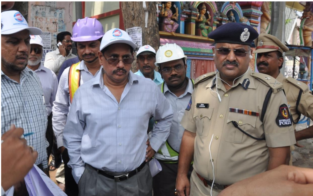
MD, HMR Mr. NVS Reddy along with Addl CP (Traffic), Mr. Jitender, inspecting ongoing Metro Rail works and traffic movement in Krishna Nagar
