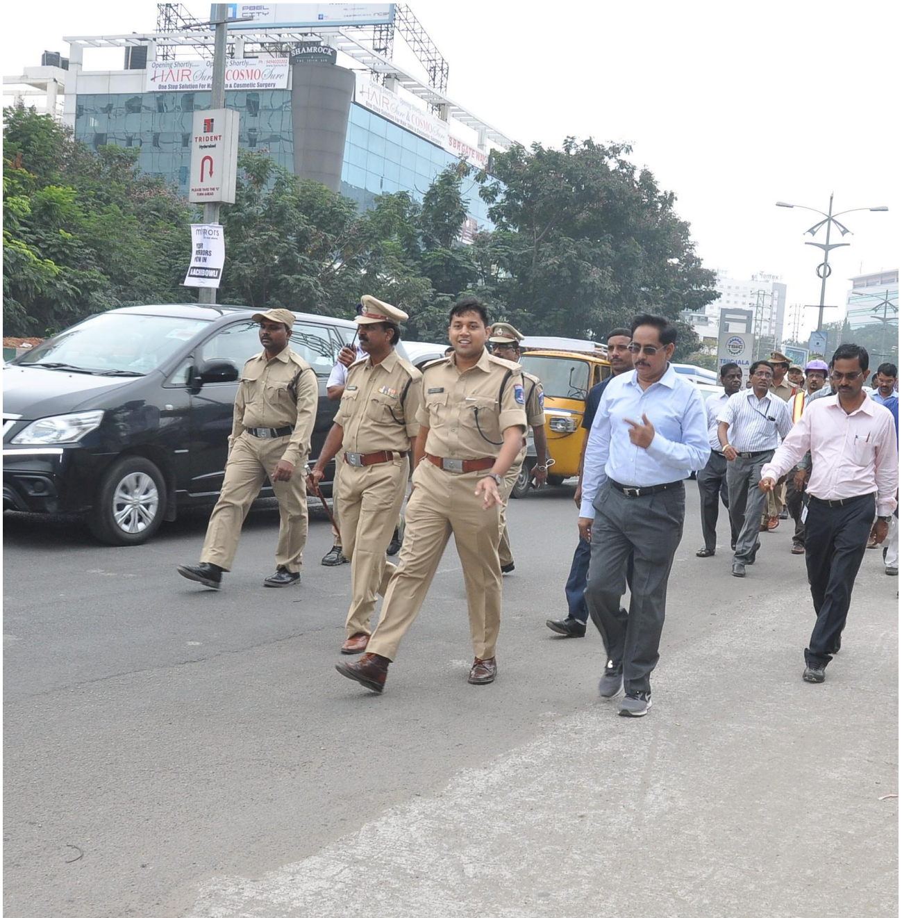
MD, HMR Mr. NVS Reddy along with DCP (Traffic), Cyberabad Mr. Avinash K Mohanty inspecting RoW alongside Metro Rail works in Hitec City today (November 21, 2015)
