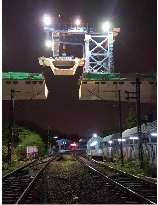
Malakpet Metro ROB under construction over the Railway tracks and Railway station using 'Bridge Builder'
