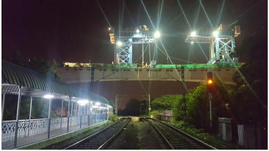
Malakpet Metro ROB under construction over the Railway tracks and Railway station using 'Bridge Builder'
