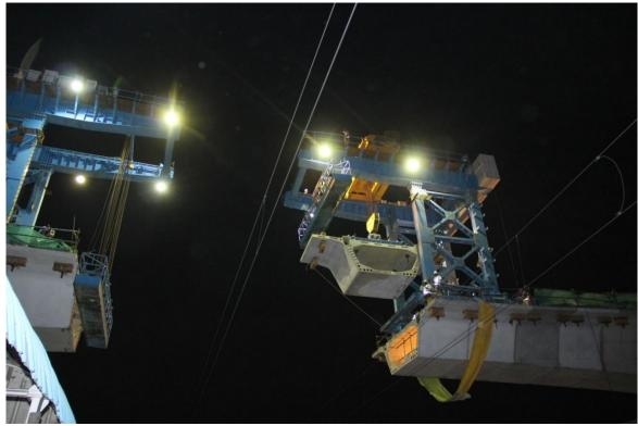
Pre cast Segment being lowered and anchored to the existing end of the viaduct at Malakpet ROB
