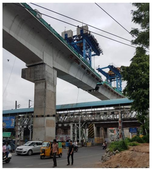
Malakpet Metro ROB under construction over the Railway station using 'Bridge Builder'
