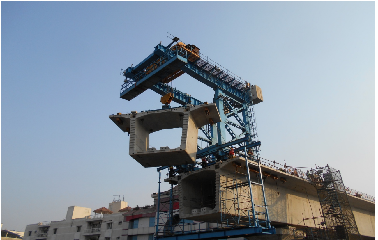
Launching of precast segment in the construction of Begumpet Metro ROB
