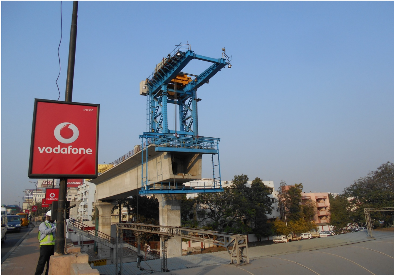
Anchoring of 'Bridge Builder' in the construction of Begumpet Metro ROB
