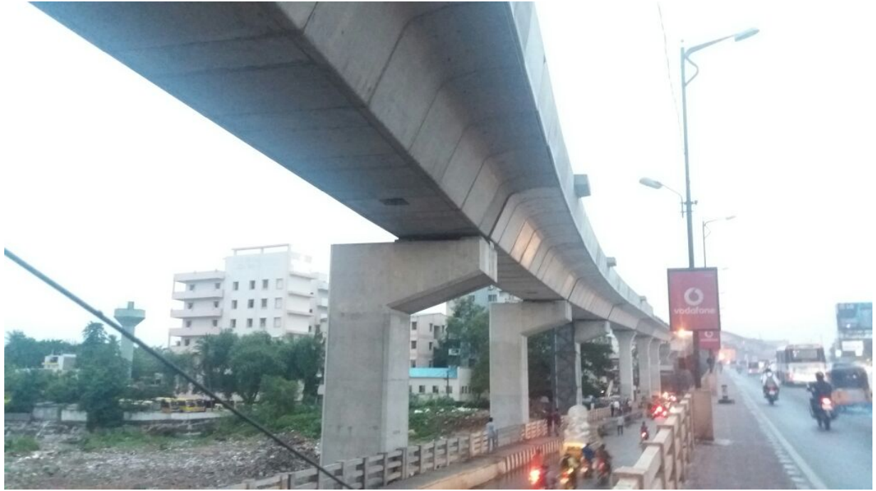
Completed view of Begumpet Metro ROBusing Bridge Builder,parallel to the existing flyover
