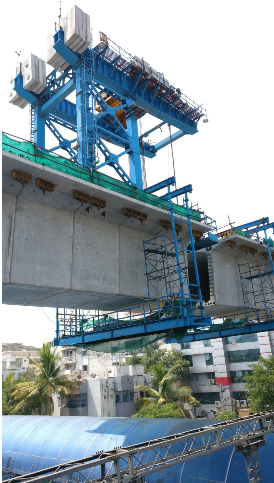
Begumpet Metro ROB construction using specially designed 'Bridge Builder'
