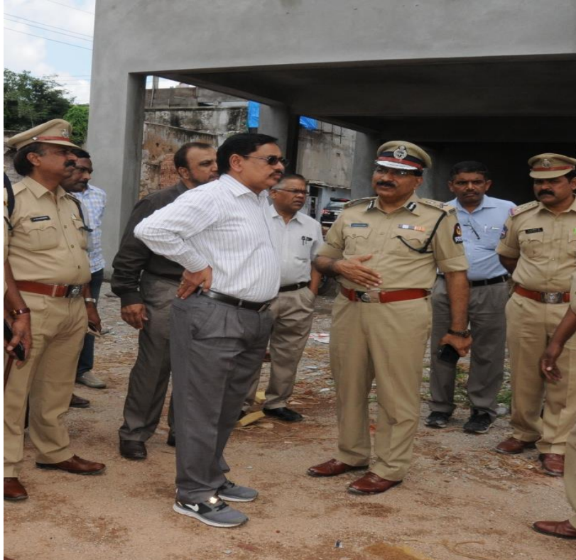
MD, HMRL Mr. NVS Reddy and Commissioner of Police, Hyderabad Mr. M. Mahender Reddy inspecting the construction works of Police barracks at Chelapura on Friday (July 29, 2016)
