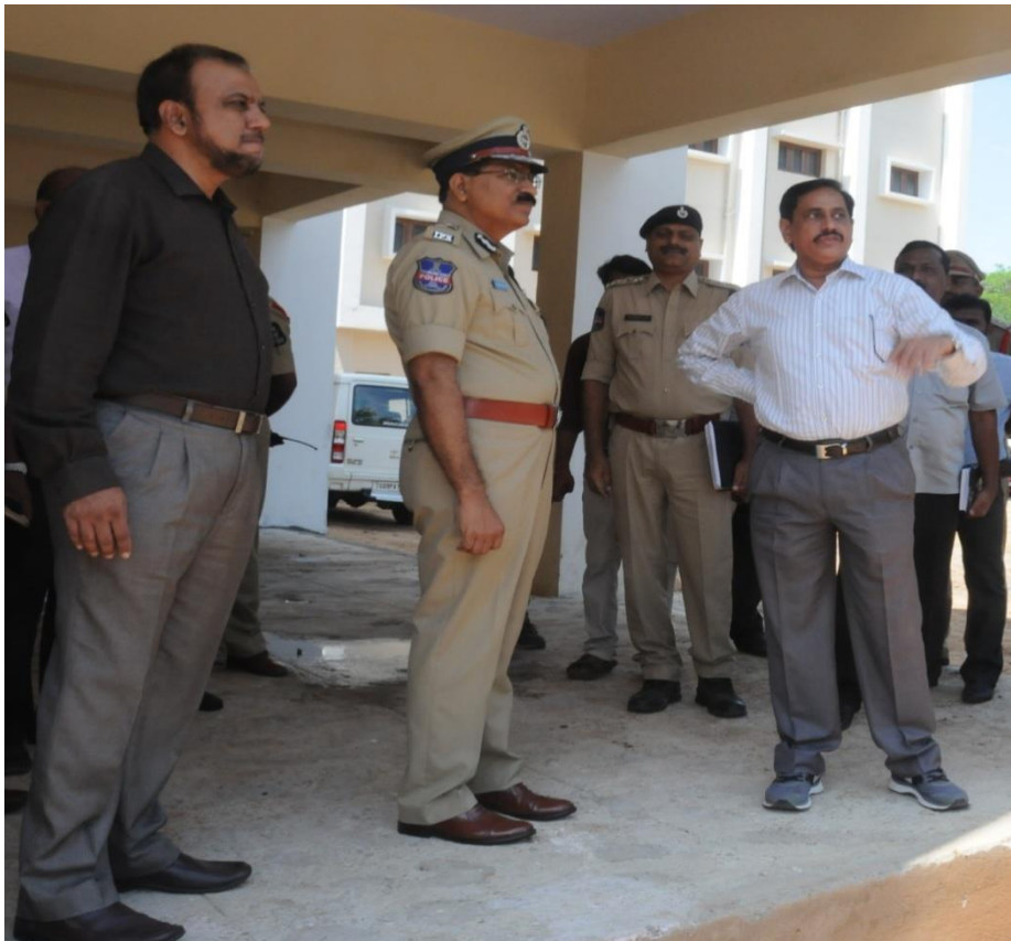
Commissioner of Police, Hyderabad Mr. M. Mahender Reddy and MD, HMRL Mr. NVS Reddy inspecting the construction works of Police barracks at Goshamahal on Friday (July 29, 2016)
