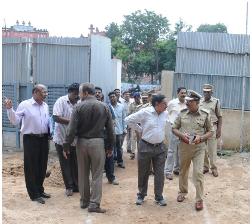
MD, HMRL Mr. NVS Reddy and Commissioner of Police, Hyderabad Mr. M. Mahender Reddy inspecting the construction works of Police barracks at city college on Friday (July 29, 2016)
