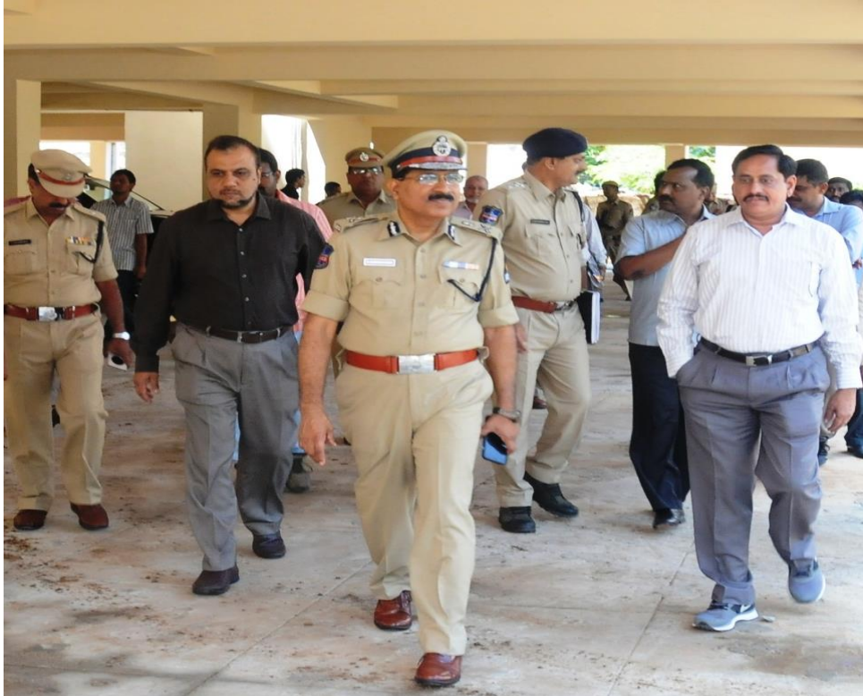
Commissioner of Police, Hyderabad Mr. M. Mahender Reddy and MD, HMRL Mr. NVS Reddy inspecting the construction works of Police barracks at Goshamahal on Friday (July 29, 2016)
