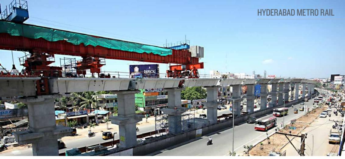
Launching Girder - State of the art construction equipment used to build elevated viaducts of Hyderabad Metro Rail
