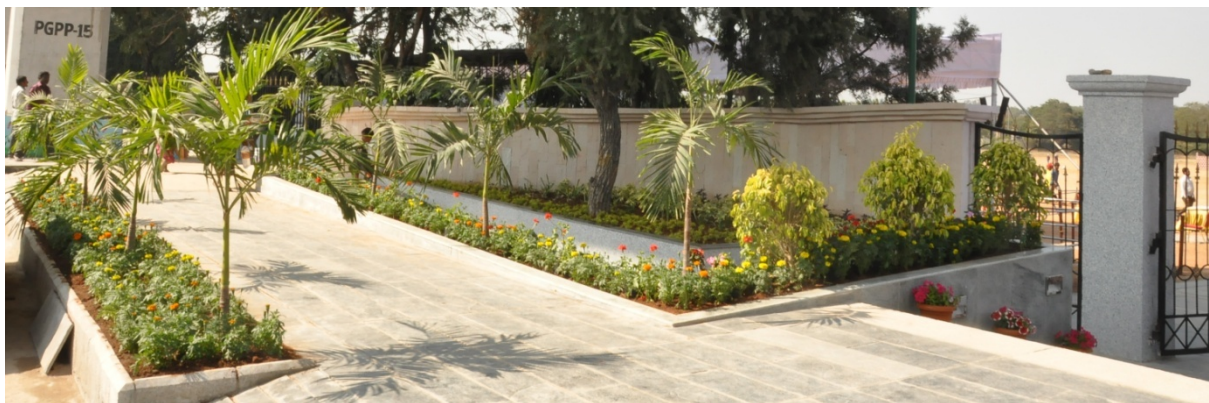
Beautification and pedestrian facilities developed by HMR at Parade grounds
