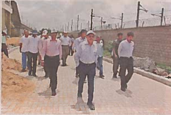
ON DUTY: NVS Reddy inspecting the ongoing urban rejuvenation works at different Metro stations between Miyapur and SR Nagar.
