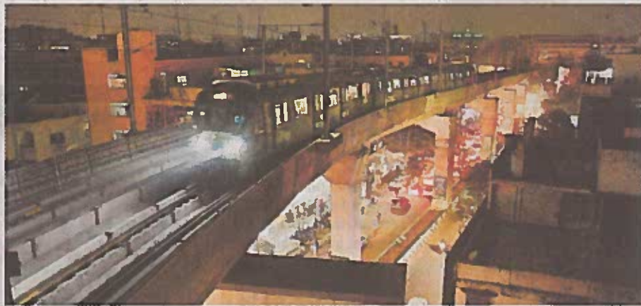
Hyderabad Metro Rail passing through the Begumpet stretch on Monday night. ■ NAGARA GOPAL
