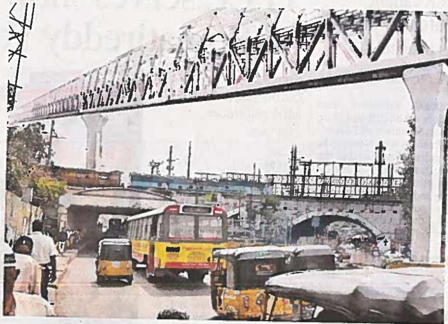
AWAITED: The bridge over the Oliphant railway bridge will be completed in January next year.
